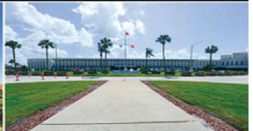
USSOCOM Command Group SCIF Project USSOCOM Headquarters MacDill AFB Tampa, FL
